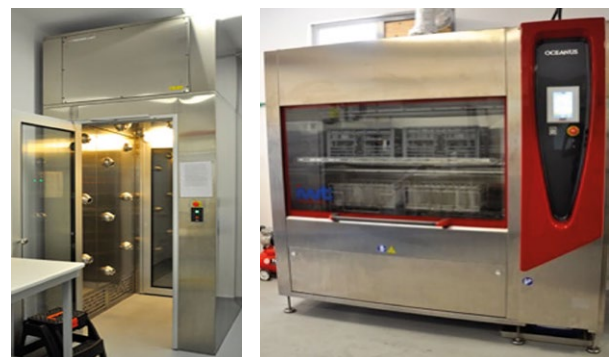
i) Genome Editing Lab ii) Cage/bottle washer iii) Air shower unit
